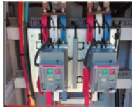
DSE ABB CHANGE OVER DEEP SEA CONTROLLER
