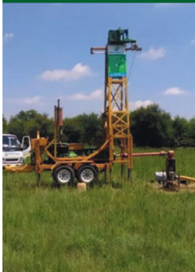
Borehole Cleaning & Rehabilitation
